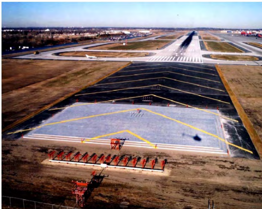
FIG AD 1.1-56 Engineered Materials Arresting System (EMAS)
